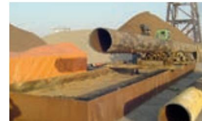
Once the topside module is confirmed as clean, salvageable equipment and components will be removed from the topside. Modules may be cut and segmented using a combination of shears and burn torches to a transportable size at the yard or shipped in bigger pieces to a scrap yard for final reduction.
