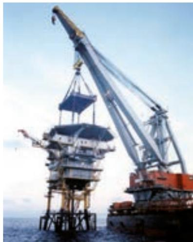
Most topsides can be lifted using a four point/single hook lift arrangement, without the use of a spreader frame/spreader beam in the same manner as the original installation method. Alternatively a spreader can also be used as determined by the contractor, reducing the horizontal forces in the top deck of the module.
