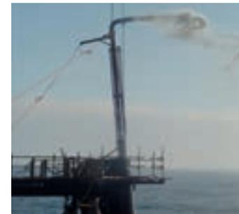
For internal cutting, the soil level should be a minimum of 2m below the required cutting elevation to allow for clearance for the cutting tool and to allow for soils entering the pile through the abrasive jet cut. The removal of the soil plug is usually done by means of airlifting. Here an airlift string is stabbed inside the pile with the HLV crane. By inserting air at the mouth of the pipe, water and sand are evacuated to the top of the pile at jacket top level.
