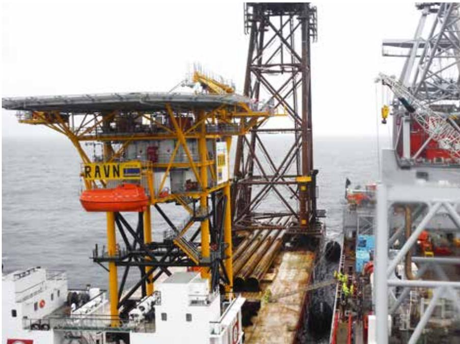
The Oleg Strashnov successfully installed the RAVN platform last May. The platform and piles were transported by the cargo barge Boa 36 to the offshore location.
